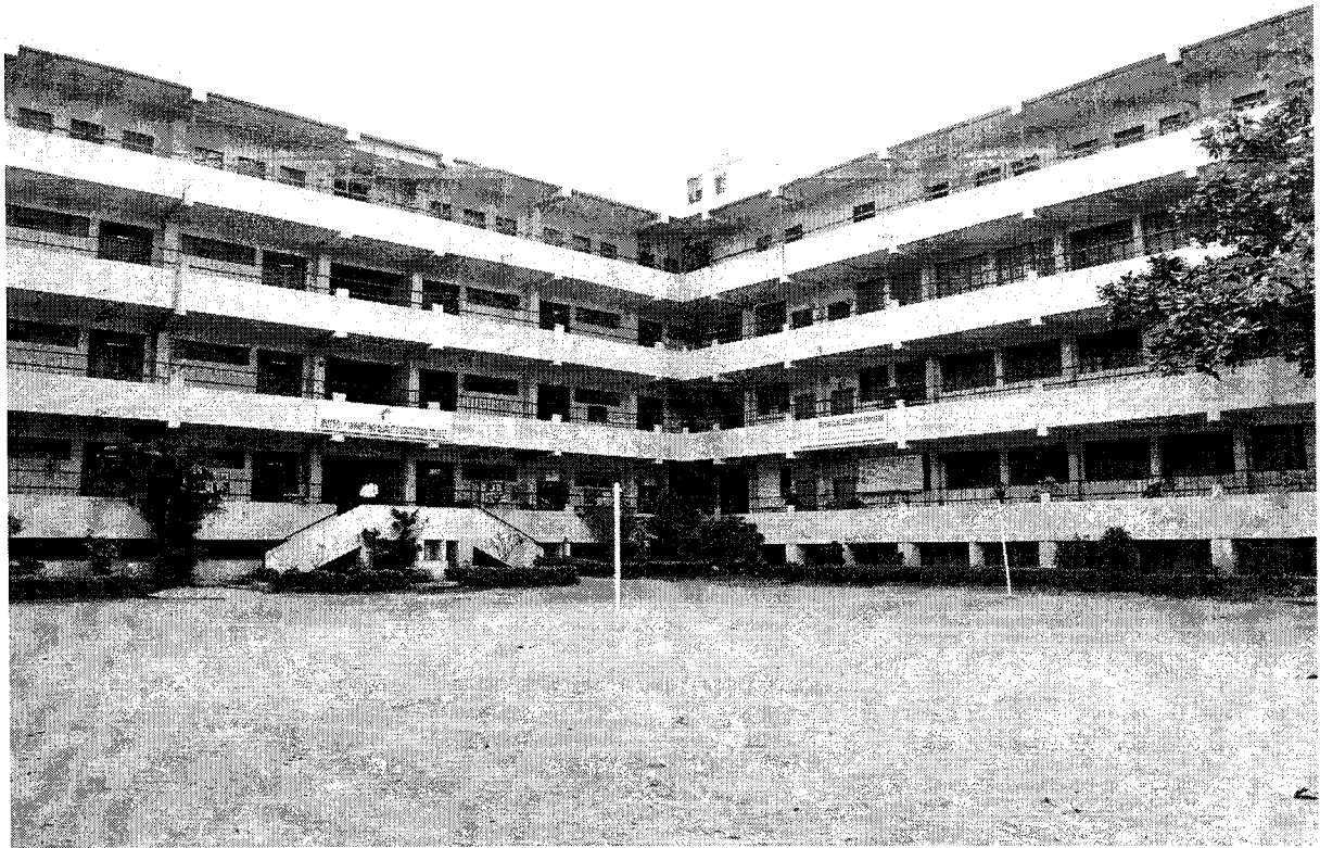
Rear view of the building
